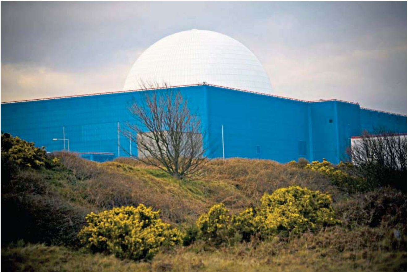
Sizewell B in Suffolk. It is questionable that we should tie into nuclear sites until 2080 to support a submarine deterrent that may be obsolete in 10 years
