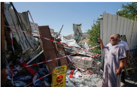
The shop after being demolished
