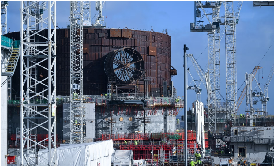
Hinkley Point C in construction
